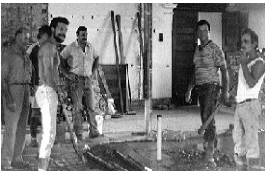
Photo: of the Ikarian Brotherhood members and volunteers during Ikaros Hall renovations.
