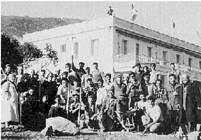
Construction of Ikaria's Hospital Άγιος Κύρικος
